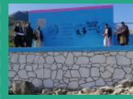
A solar-powered water supply network handed over in Kunar province ...
