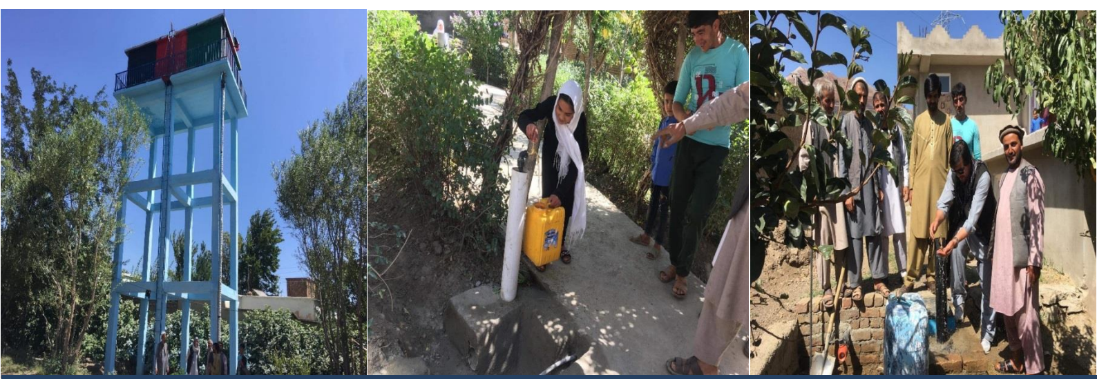
The newly-constructed water supply network in “Eshq Abad” village in Jabal Seraj district of Parwan province
