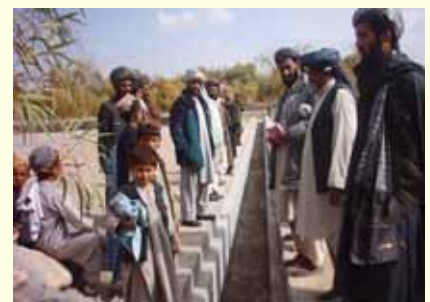
Canal construction project: Increasing productivity of agriculture
