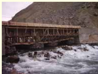
Worsaj Bridge in Worsaj, Takhar Province is being constructed in June 2005.
