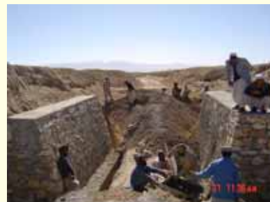
Construction of a wash culvert in Ander Dist, Ghazni province in October 2004.
