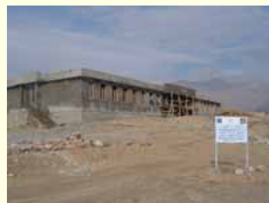
Alikheel School being constructed Deh Sabz, Kabul, November 2004.
