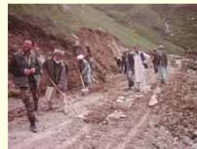
Construction of the road in Yaftal Yawan, Badakhshan Province in 2005.
