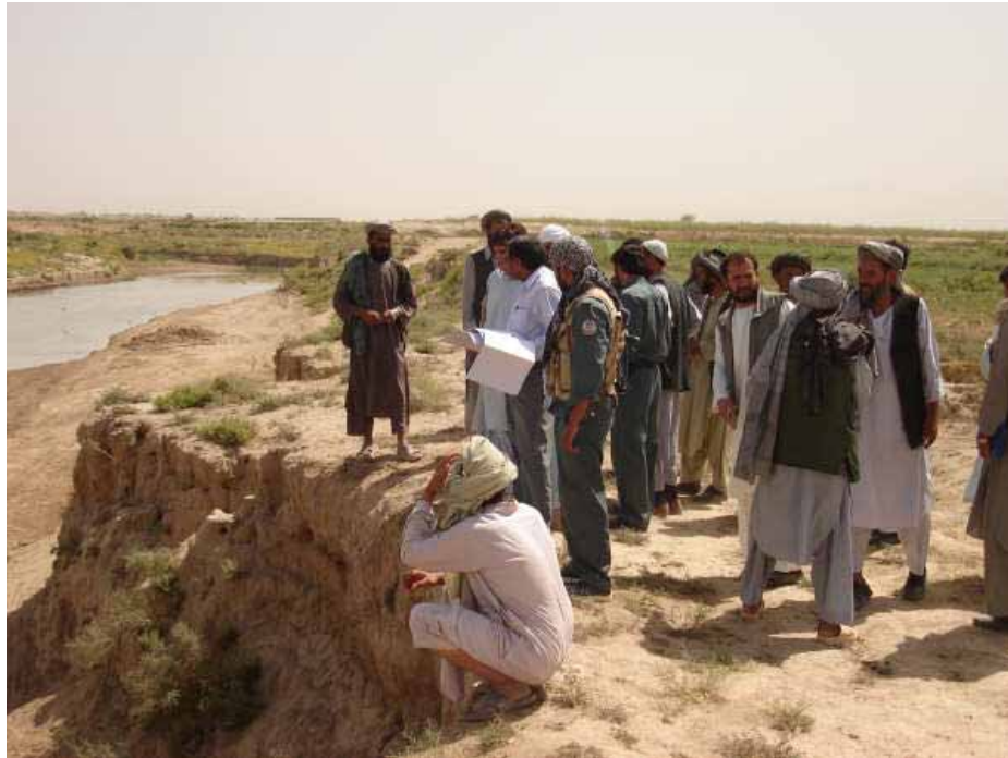
Technical Assessment at the construction site of the Chimtal Bridge in Balkh Province
