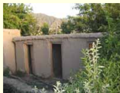
Latrines constructed in Dand Patan district, Paktia Province.
