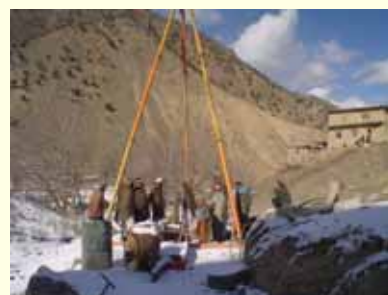
Drilling a well in Lajamangal district, Paktia Province.
