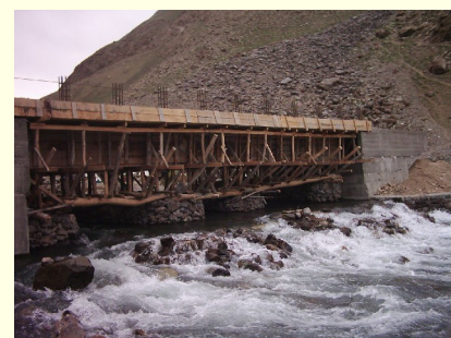
Worsaj Bridge in Worsaj, Takhar Province constructed in June 2005.
