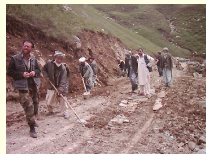
Construction of road in Yaftal Yawan, Badakhshan Province in 2005.
