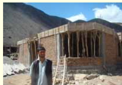
Panjsher Directorate of Rural Rehabilitation and Development building is under construction.
