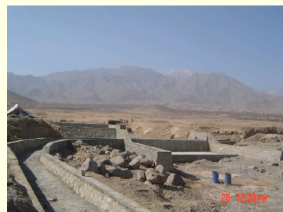
Wash culvert constructed in ash Shakardara, Kabul, November 2004.
