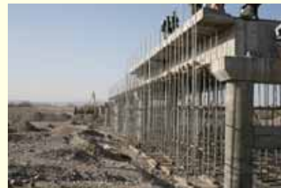
A 180-meter long bridge on Arghandab River in Kandahar is under construction by MRRD's National Area-Based Development Programme, the funding of which has been provided by CIDA.
