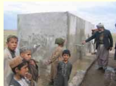
A piped water system was constructed in Buldak District, Kandahar Province, 2005.
