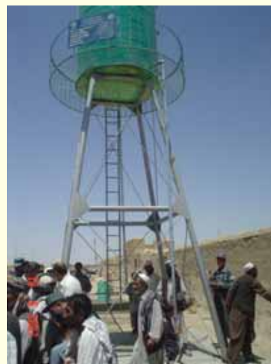
Completion of the Construction work of a 10,000-liter water reservoir in Aqcha District of Jawzjan Province
